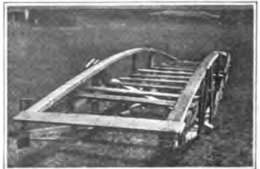
BOWSTRING SPAN COMPLETE BUT FOR FLOOR-BOARDS
